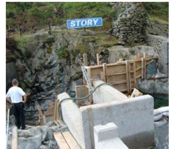
Further developments during construction of intake
