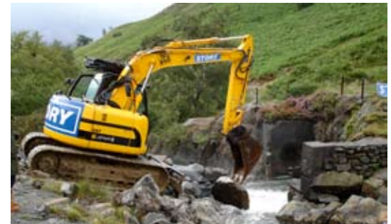
Work starting on intake
